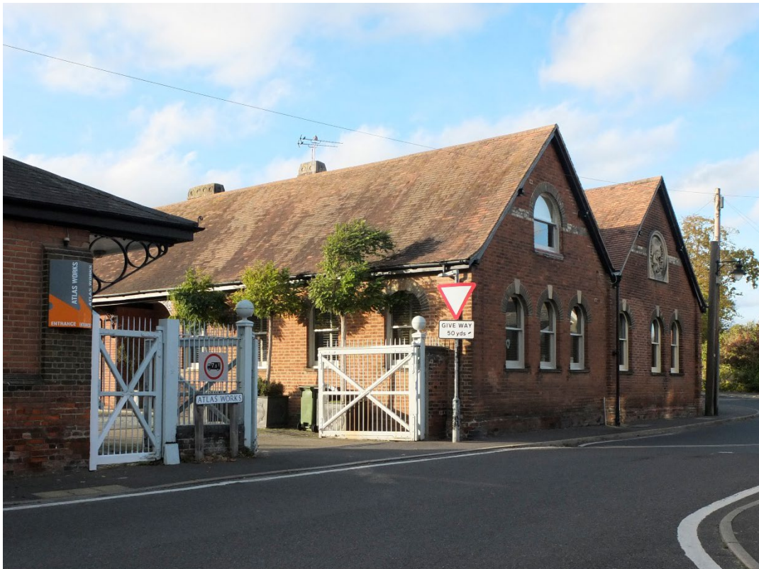
Atlas Works in Earls Colne Conservation Area
