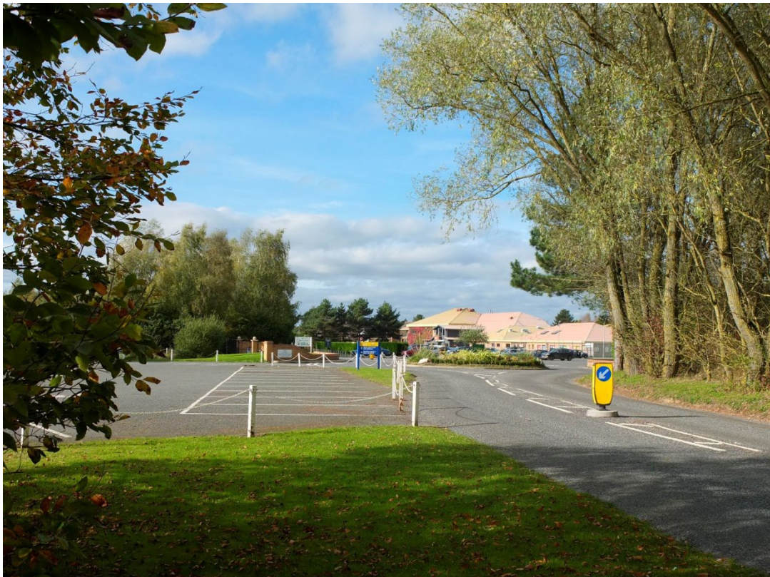
Business Park at Earls Colne Airfield
